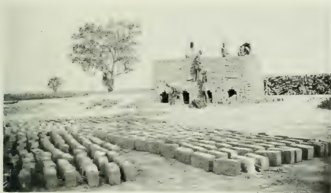
BRICK MAKING. THE FIRST KILN IN WAU.
